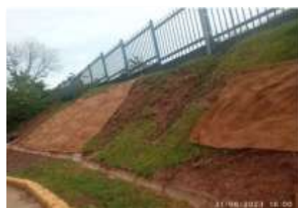
Revegetation of embankments. Panama. August 2023. Hydraulic Infrastructure.
