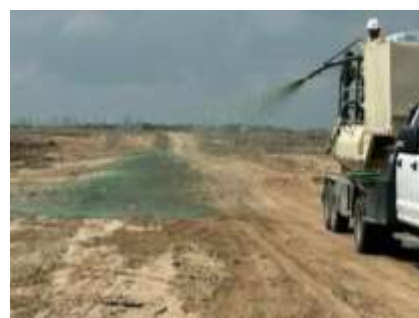
Hydroseeding. SWPPP. United States. Photovoltaic infrastructure. March 2023.
