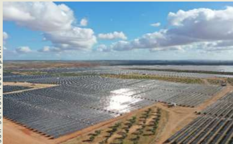
ENERGY San Serván 400. Spain
