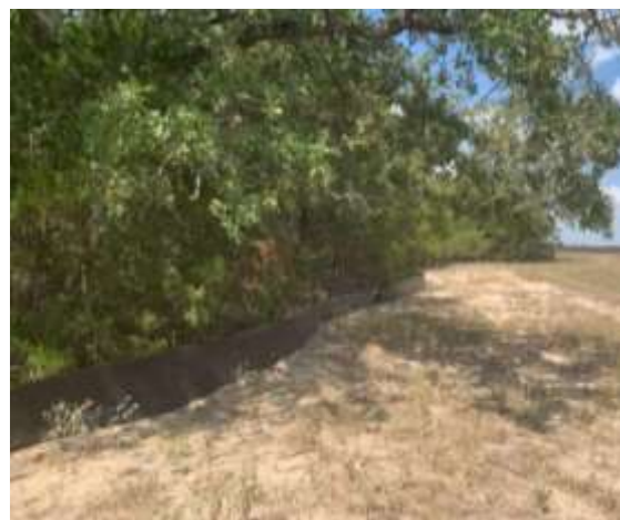
Best Practices. Protection of waters: erection of silt fences. September 2022
