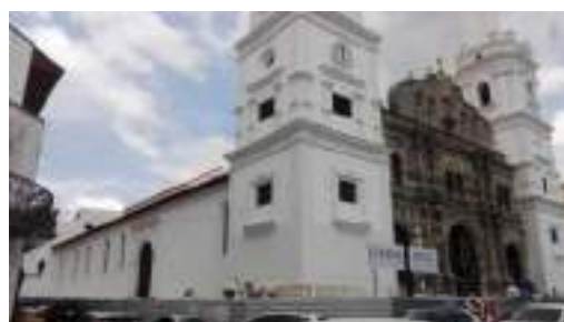
Restoration of St. Mary's Cathedral (Panama City)
