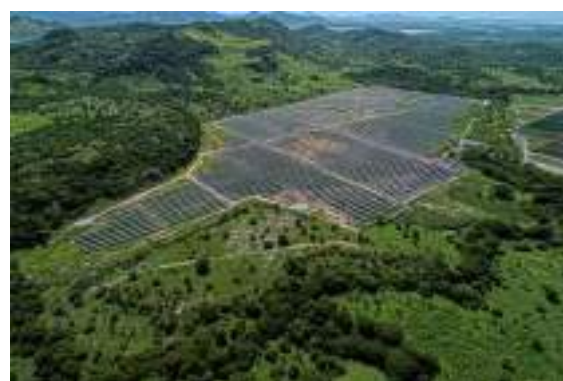
Photovoltaic solar plant in Aguascalientes (Mexico)
