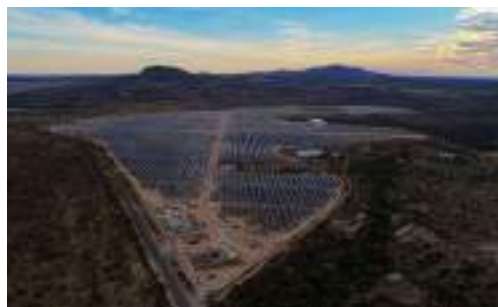
Mexico Photovoltaic plant
