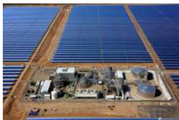
“La Africana”(50 MW) thermosolar plant in Almodóvar del Río, Córdoba
