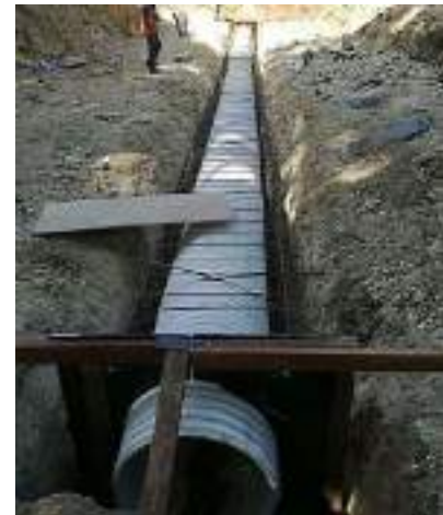
San Miguelito sewage system. (Panama)
