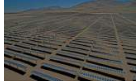
Photovoltaic plant in Honduras
